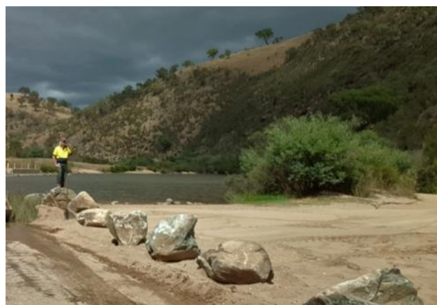
Installation of boulders to prevent vehicular access to the river at Angle Crossing (PCS)
