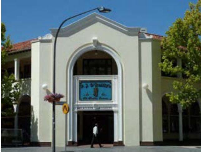
Figure 9. Solid splayed corner bay at the Alinga Street/West Row corner
