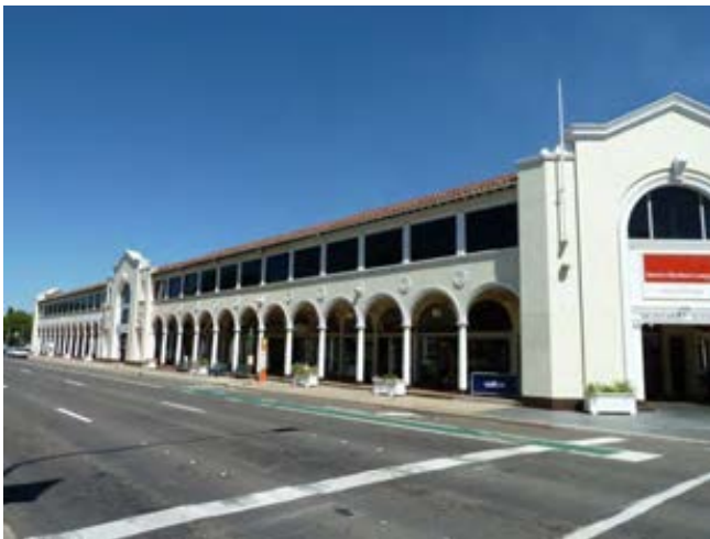
Figure 4. Eastern elevation of the Melbourne Building facing Northbourne Avenue
