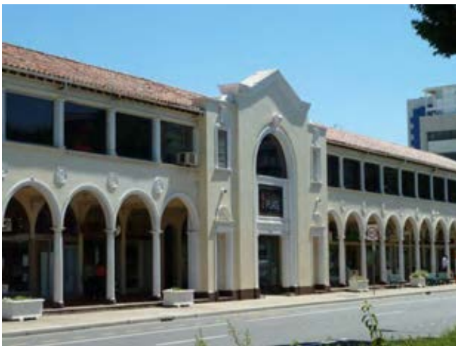
Figure 10. Section of the Northbourne Avenue colonnade of the Melbourne Building
