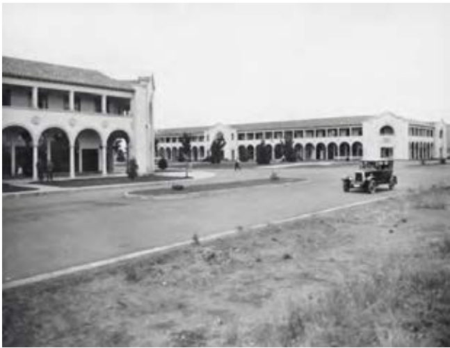
Figure 38. Sydney and Melbourne Buildings, 1938
