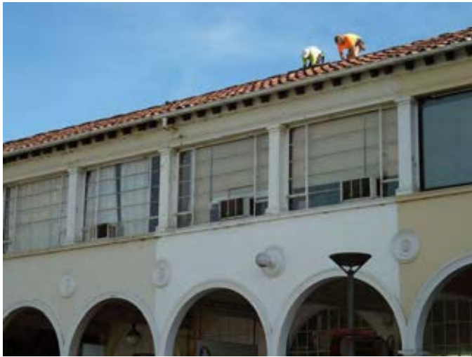
Figure 5. Detail of elevation on East Row – note different aged infill treatments for verandahs, and window mounted airconditioners
