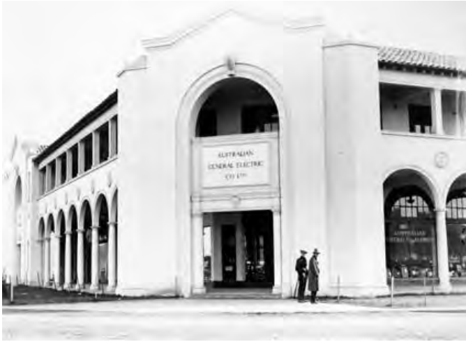
Figure 33. Premises of the Australian General Electric Co in the Sydney Building, 1928
